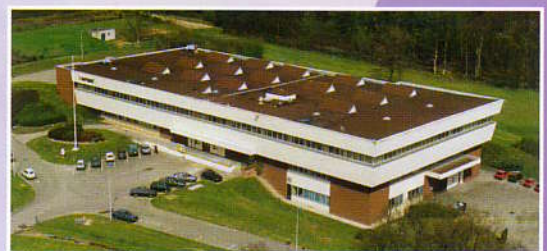
Headquarters and factory 80.700 sq. ft./ 7.500m 2
