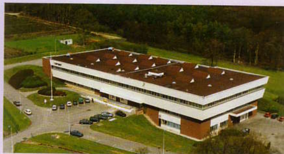
Headquarters and factory 80.700 sq. ft./ 7.500m 2
